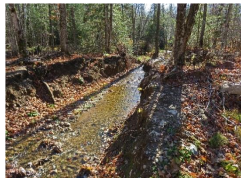
Desbarats Lakes Road Erosion and Channelization
