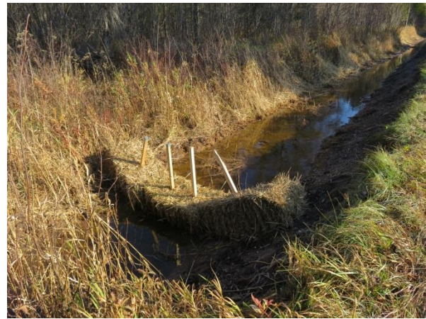
Typical Sediment Control
