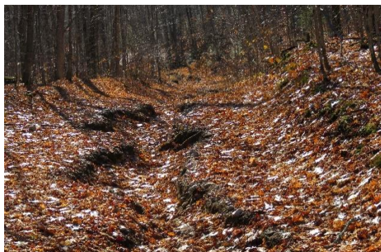
Desbarats Lakes Road Erosion and Channelization
